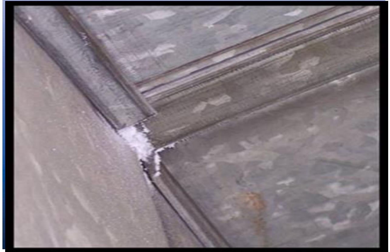
Aerosol-based duct sealing
